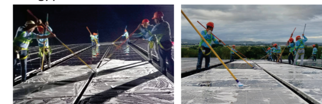
Regular Cleaning of solar panels.
