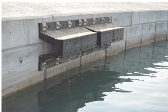
V-shaped solid fender installed on the quay wall
