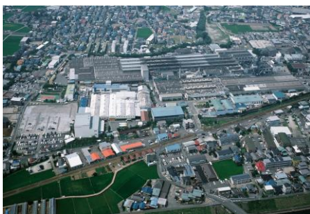
Yokohama Rubber's Mishima Plant
