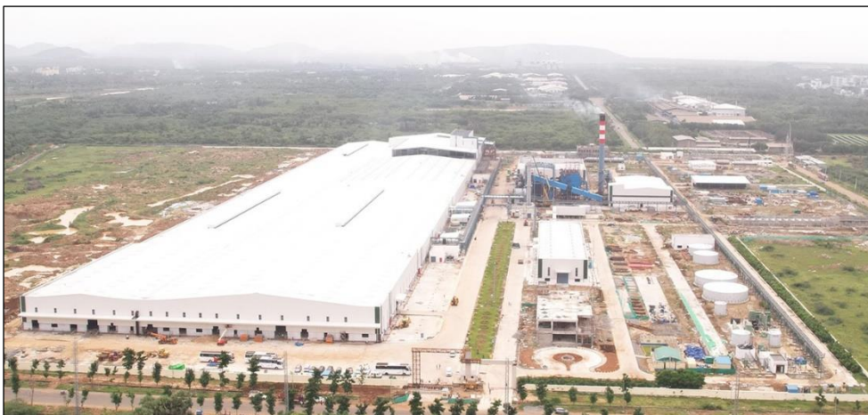
The Visakhapatnam Plant
