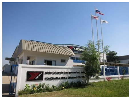
Yokohama Mold (Thailand)
