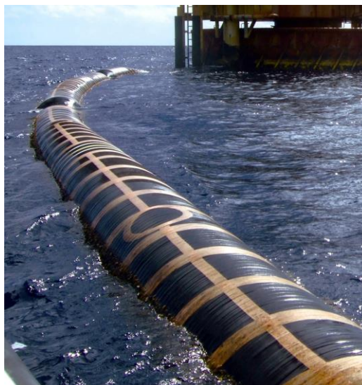
Seaflex hose transporting crude oil
