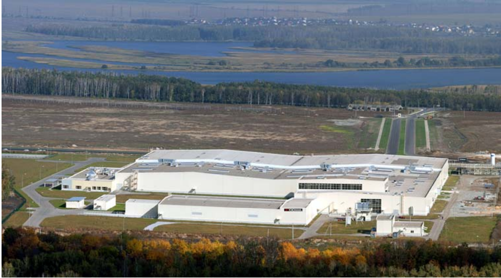
Bird-eye view of Yokohama R.P.Z.'s tire plant in the region of Lipetsk, Russia.
