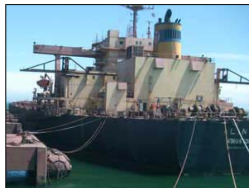
Pneumatic fenders installed between a vessel and a wharf
