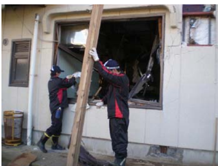
Removing debris from a building
