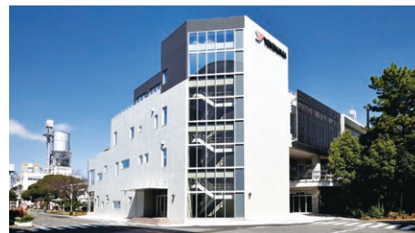
New dual purpose conference room and cafeteria in Hiratsuka
