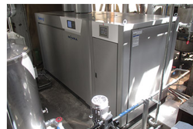
Steam driven compressor
