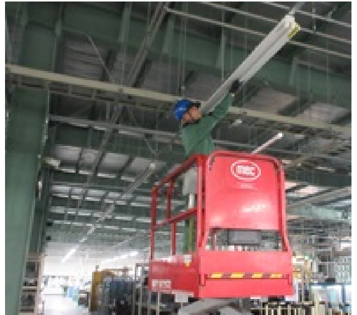
Replacement of lighting
