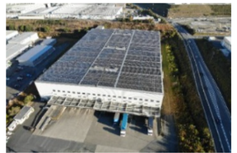
Solar power generation (Shinshiro-Minami) installed capacity : 1,040kw
