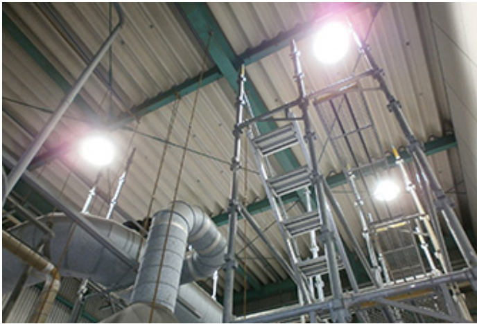
Mercury lighting → LED lighting
