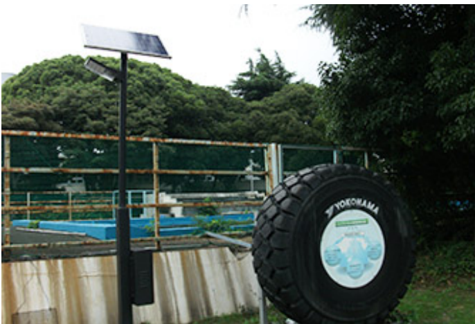
Installation of solar street lights
