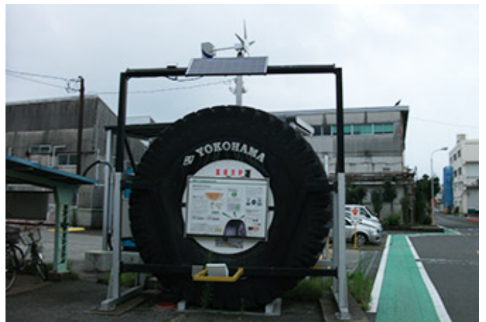
Installation of solar and wind powered street lights
