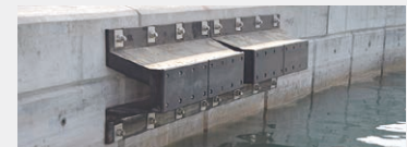
V-type solid fender installed on the quay wall
