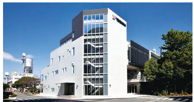
New dual purpose conference room and cafeteria in Hiratsuka
