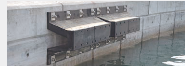
V-type solid fender installed on the quay wall
