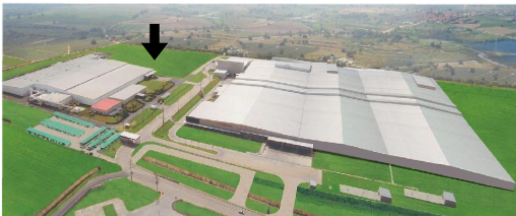
External view of the YTMT. The area indicated by an arrow is the land for constructing the second TB tire plant.
