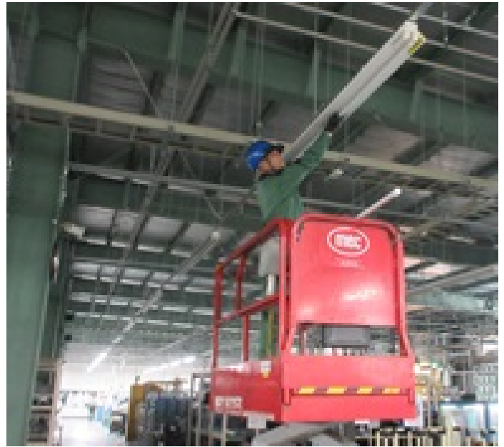
Replacement of lighting
