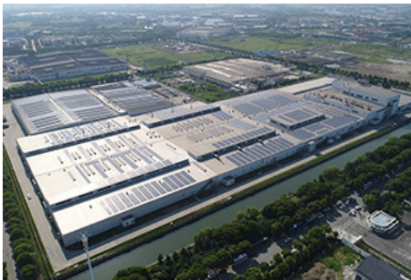
Solar power generation (Suzhou, China) installed capacity: 3,000 kw
