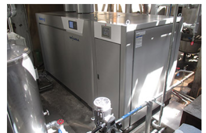
Steam driven compressor
