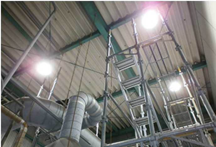
Mercury lighting → LED lighting
