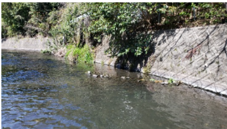
Construction of "barbed construction" in collaboration with river jurisdiction
