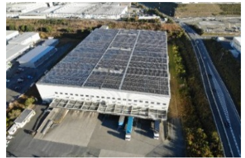
Solar power generation (Shinshiro-Minami) installed capacity : 1,040kw
