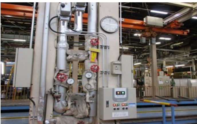
Separated the steam system and installed a motor valve
