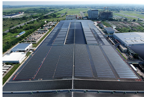
Solar power generation (Philippines) installed capacity: 4,000 kw
