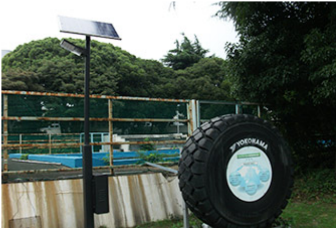
Installation of solar street lights
