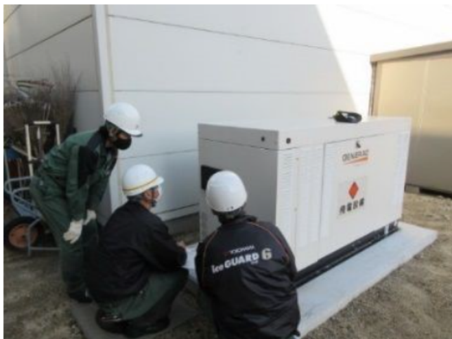
Emergency power generator inspection
