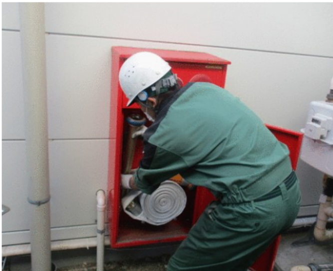
Inspection of firefighting equipment
