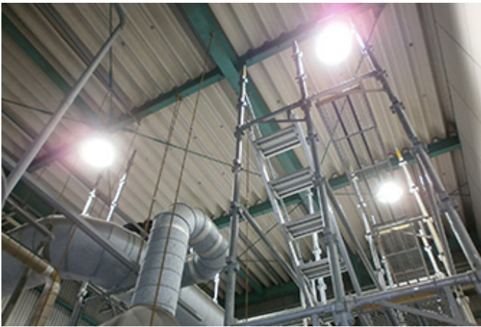
Mercury lighting → LED lighting
