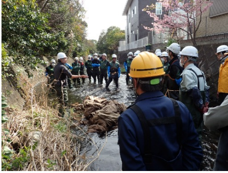
Construction of "barbed construction" in collaboration with river jurisdiction
