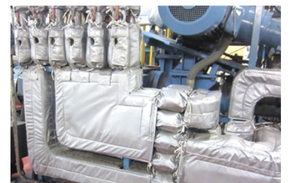
Pipe insulation
