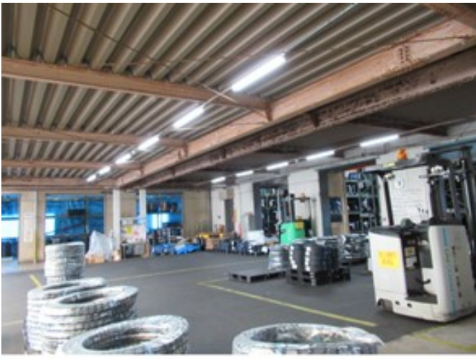
Conversion to motion sensors and LEDs
