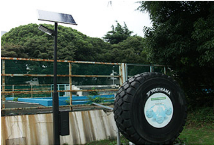
Installation of solar street lights
