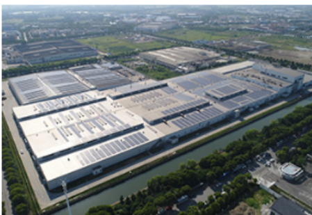
Solar power generation (Suzhou, China) installed capacity: 3,000 kw
