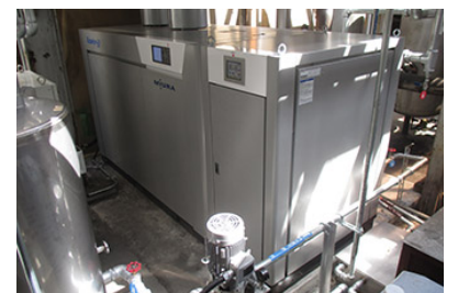
Steam driven compressor
