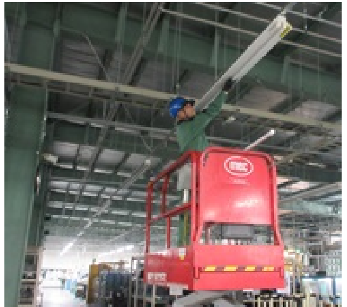
Replacement of lighting
