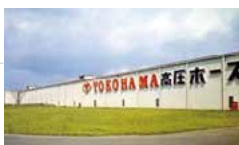
In 1974, commenced production of high-pressure hoses at the Ibaraki Plant.
