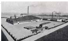
In 1920, completed construction of the Hiranuma Plant, the company's first production facility.
