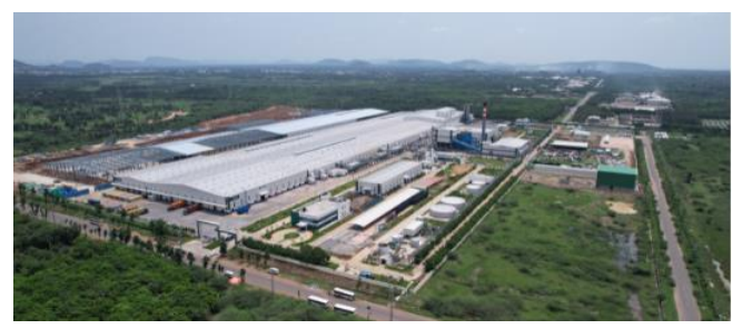
Visakhapatnam Plant, India (new wing under construction on left)
