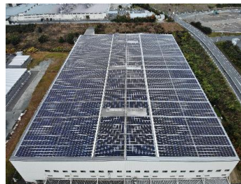
Shinshiro-Minami Plant's solar power generation facility
